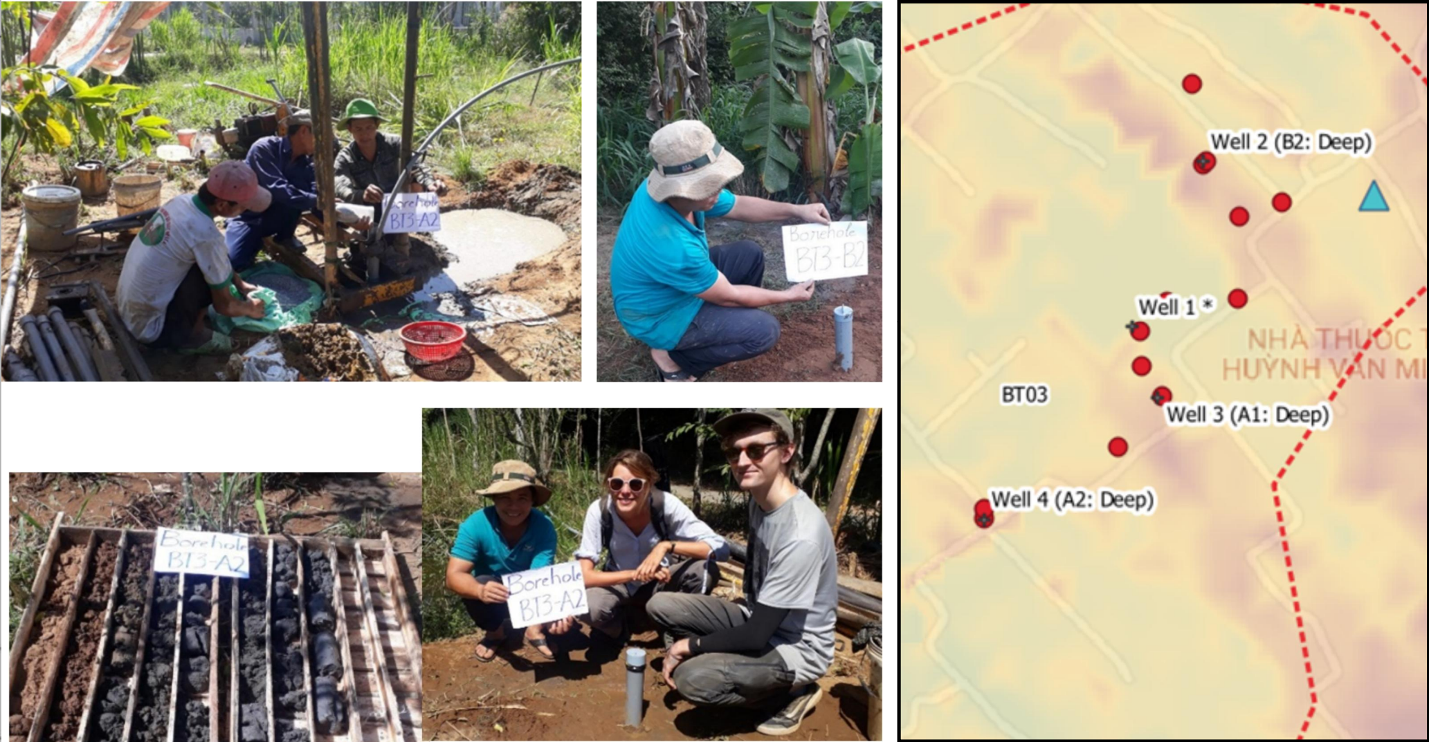
Drilling and installing the groundwater monitoring wells at BT03
