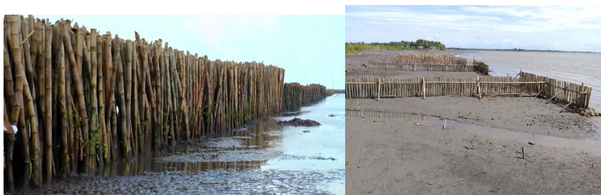
Figure 44. Permeable bamboo fences and T-groynes (Mekong Delta, Vietnam)
