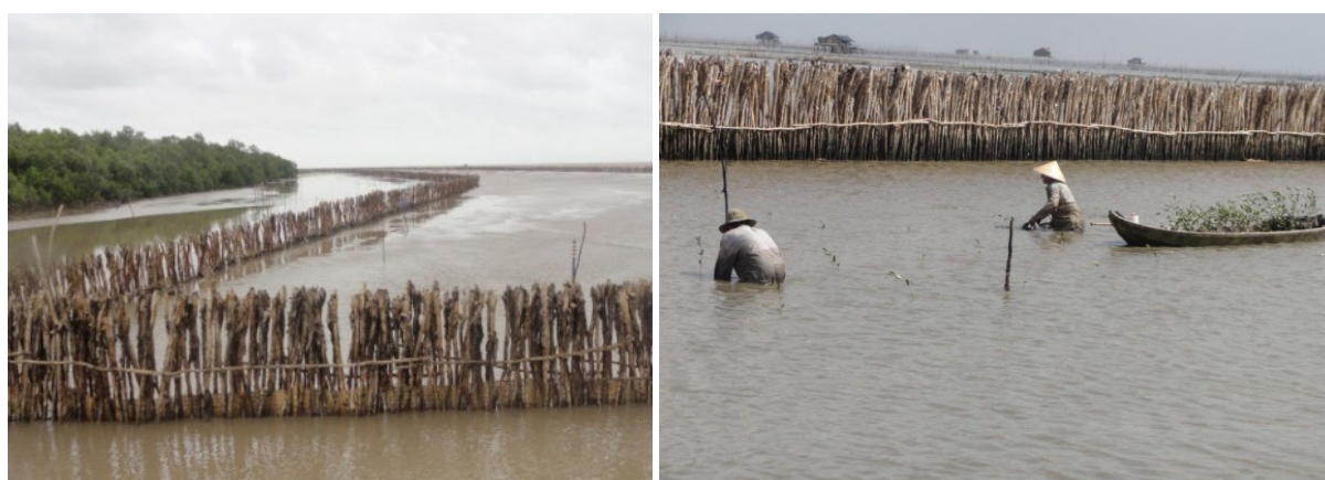
Figure 40. Mangrove planting behind bamboo/wooden fences along the Mekong Delta
