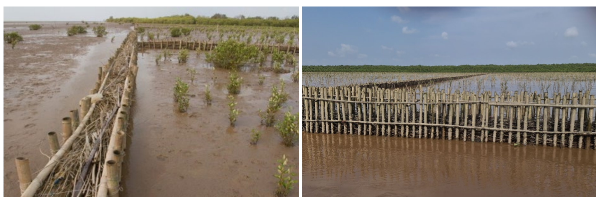
Figure 43. Mangrove rehabilitation behind bamboo fencing in Soc Trang and Bac Lieu provinces
