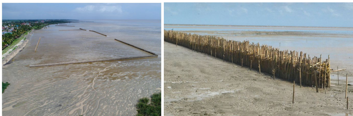
Figure 4. Permeable groynes (constructed from bamboo and brushwood) along the Guyana coast
