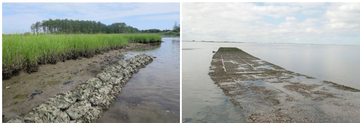
Figure 31. Examples of hybrid engineering: oyster reefs and saltmarshes in Australia (left) and oyster reefs and seagrass on tidal flats in the Netherlands (right)
