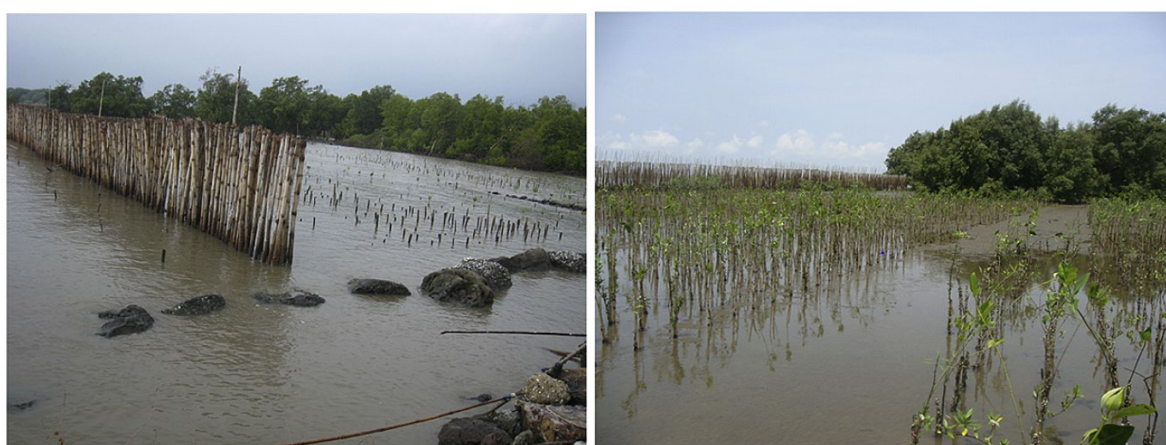
Figure 6. Bamboo fencing and successful mangrove planting behind such fences along an eroding shoreline at Chachoengsao Province (Thailand)
