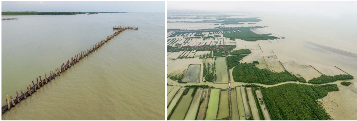
Figure 8. Successful mangrove restoration along an eroding coast at Demak in Java (Indonesia) using permeable groyne structures to trap sediment
