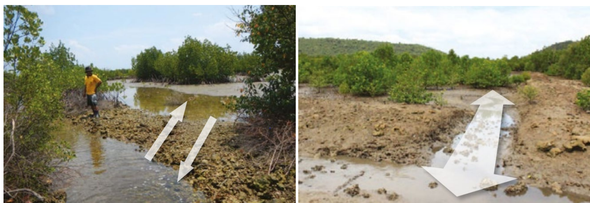
Figure 18. Small dyke preventing drainage (left) and creation of a breach to restore normal tidal hydrology (right)
