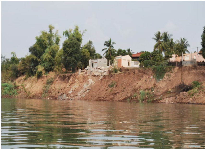
Figure 73. River bank erosion in the MD as a result of sand mining (photo Kackney et al., 2020)
