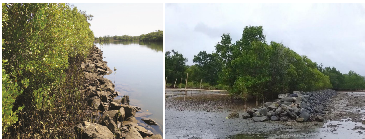
Figure 30. Examples of hybrid engineering: mangrove-breakwater combinations in Australia (left) and Philippines (right)
