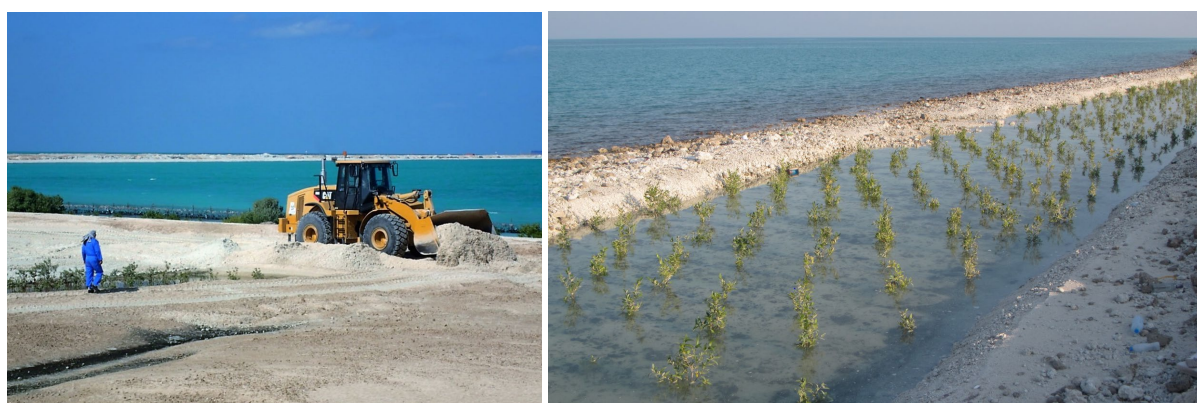
Figure 11. Mangrove planting inside artificially created tidal channel along a shoreline, temporarily protected from the sea by a berm of dredged material, to offer the newly planted mangroves time to establish and develop into a more mature stand that can function as a protective green belt against erosion (Abu Dhabi, UAE)
