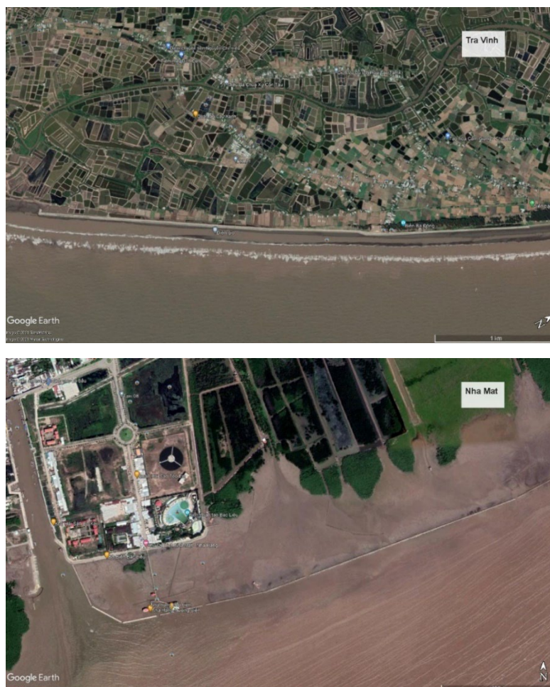
Figure 87. Example of a concrete seawall in Tra Vinh province (upper panel) and of a detached breakwater at Nha Mat (Bac Lieu province, lower panel).
