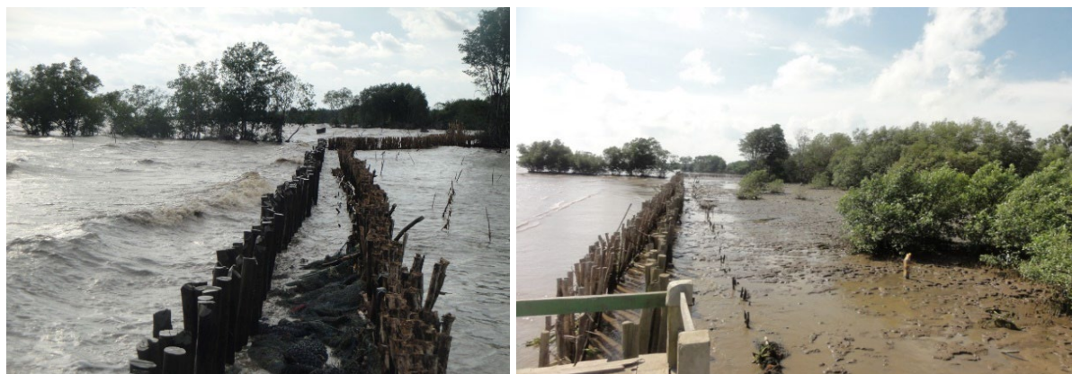
Figure 41. Mangrove rehabilitation involving Melaleuca and Eucalyptus fences in Kien Giang province to reduce wave energy and cause sediment accretion
